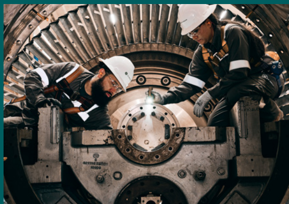
Expert craft professionals inspect a 7F gas turbine at GE Vernova's Houston Learning Center in Texas
