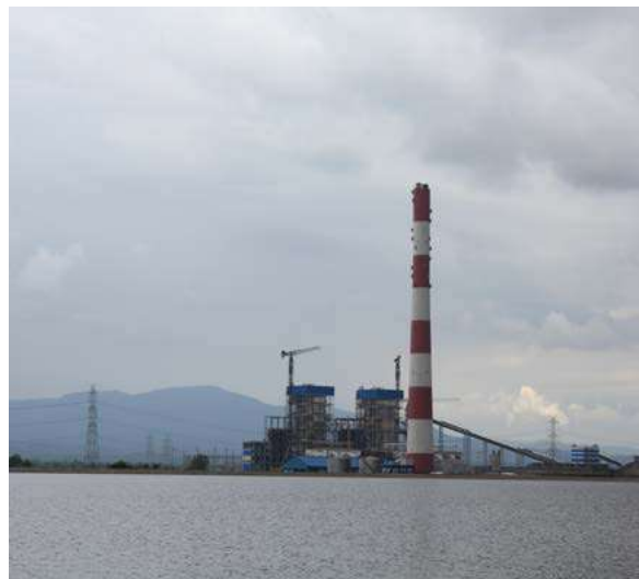
MB Power's Annupur power plant
