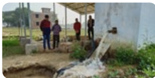
Installation of solar pump at Naini
