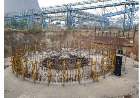
Highest ever concrete across various FGD projects
