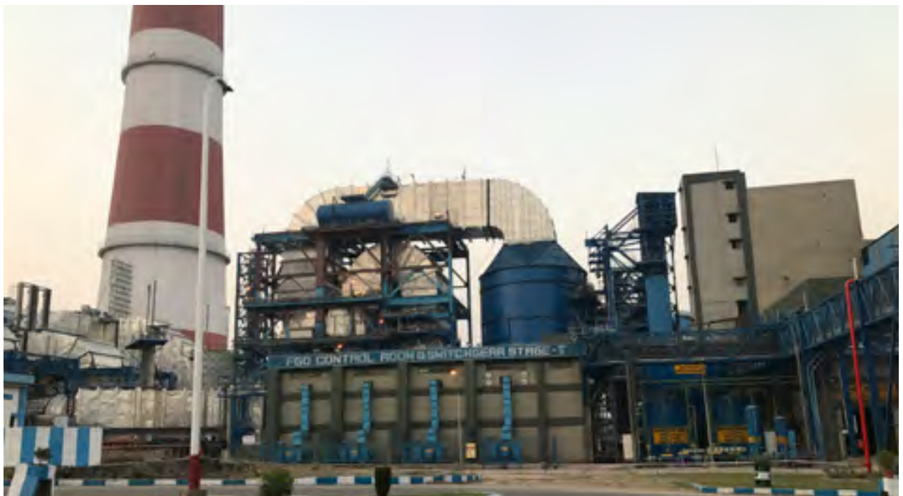
NTPC 500 MW Super Thermal Power Plant, Vindhyachal
