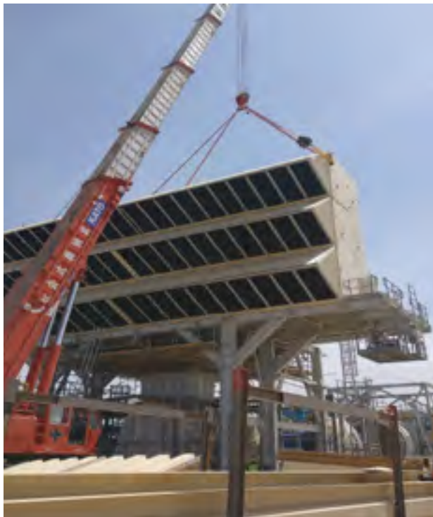
320 MW Zubair Gas Power Plant - Filter and EVAP Module Erection
