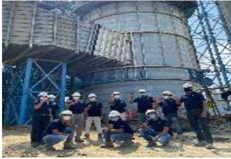
Erection of stage IV FGD absorber NTPC Unchahar WFGD plant
