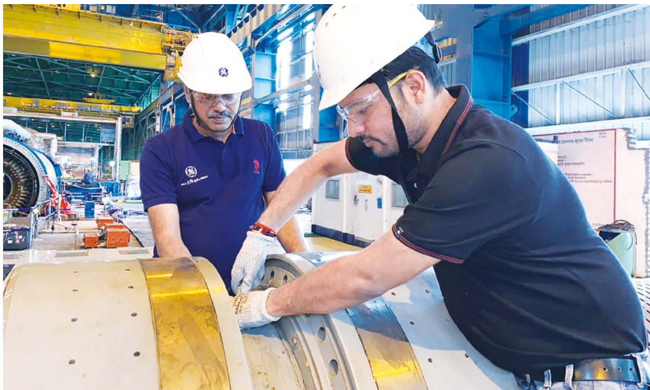
Employees working on 500MW brushless exciter servicing oOEM for NTPC Korba
