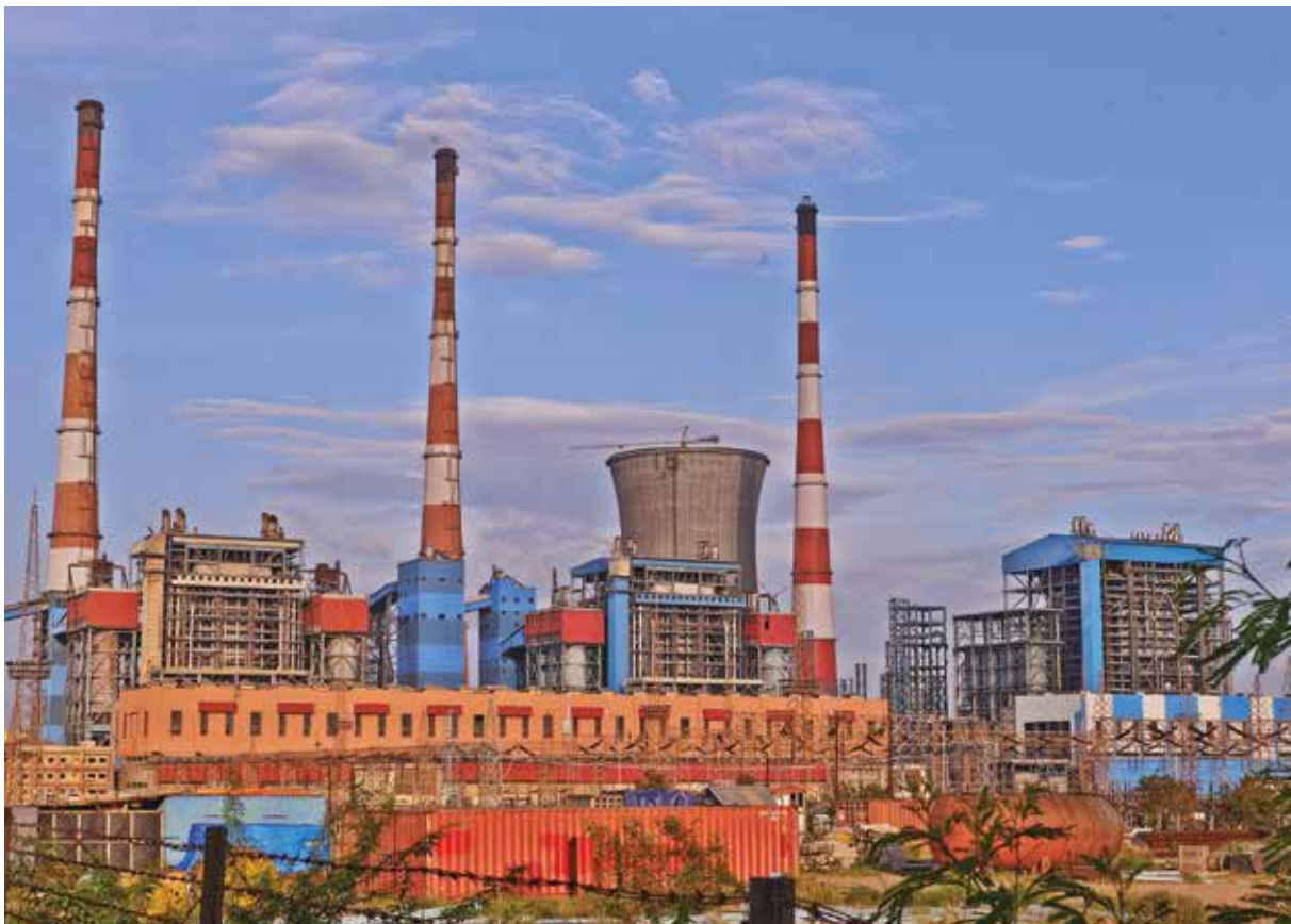
1 x 700 MW Bellary Thermal Power Station of Karnataka Power Corporation Limited
