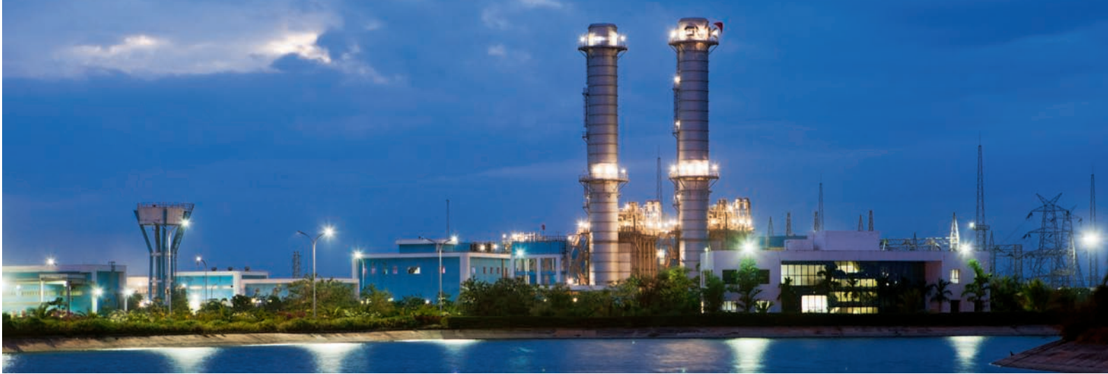
Gautami, power plant constructed by Alstom
