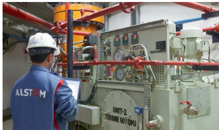
Chamera, Alstom Hydro Project Site
