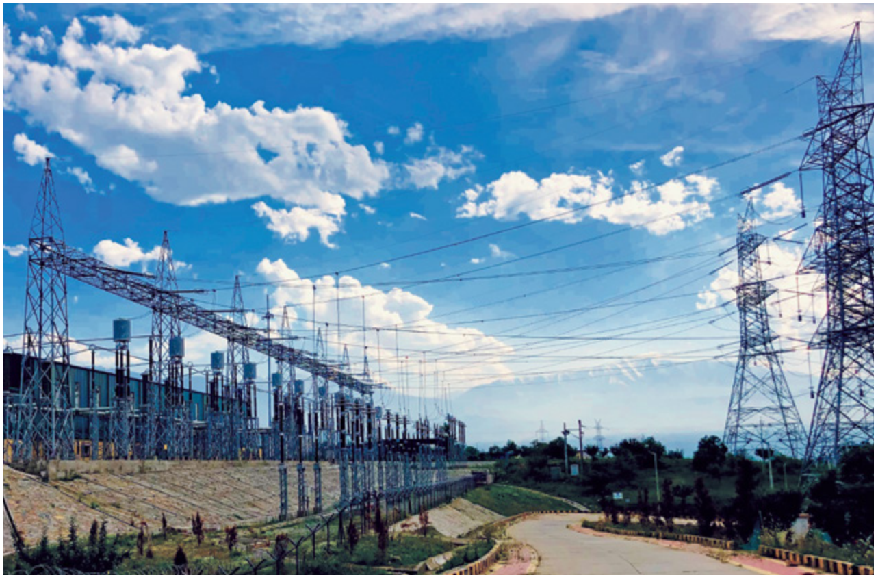
Commissioned 400/220 kV Gas Insulated Substation situated at an altitude of 2024 mts (6640 ft) in Amargarh, Kashmir
