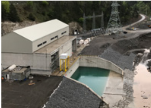
2 x 89.3MW Shuakhevi hydropower plant in Adjara, Georgia
