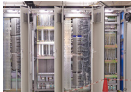
Automation and Controls office in Noida
