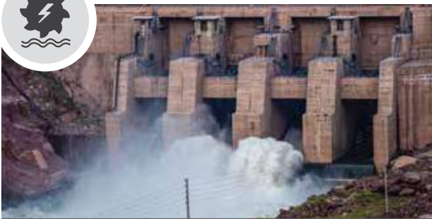
Uri Hydropower Plant, Jammu & Kashmir
