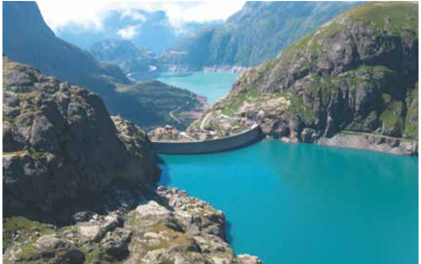
Nant de Drance Hydropower plant
