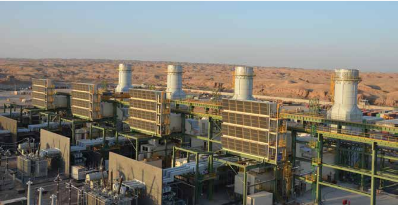
728MW Al Mansurya gas power project in Iraq
