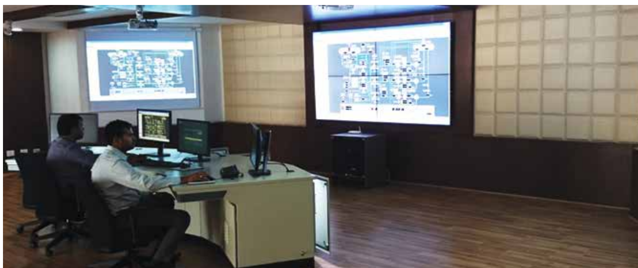
Demo and training centre at Noida Power Automation Control unit
