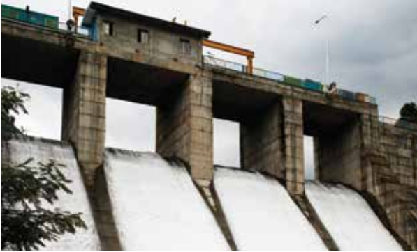
Successful commissioning of 2x55MW Chuzachen hydro-electric project
