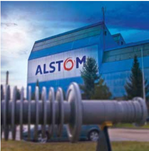
> Karlovac factory, Croatia, site overview
