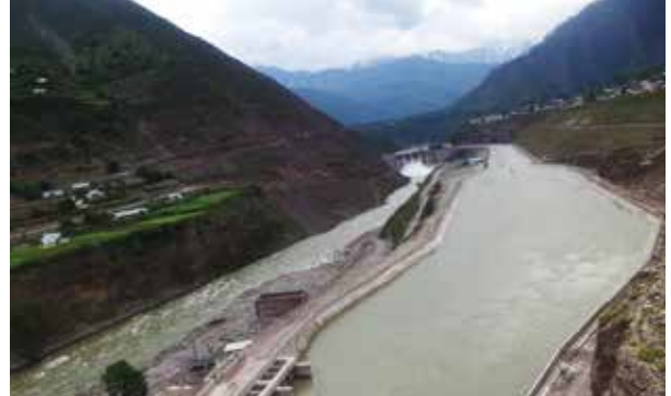
Successful commissioning of Uri II 4x60MW hydro project in Baramulla
