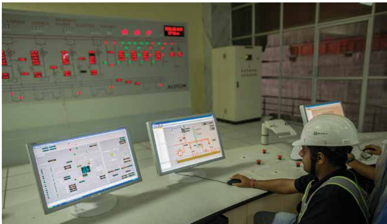
6x40MW Lower Jurala hydro project in Andhra Pradesh
