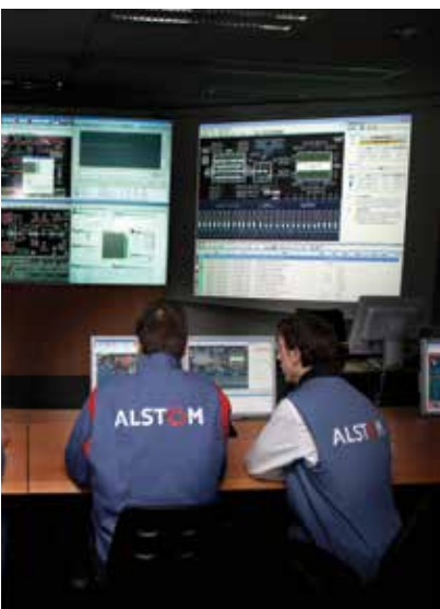
Control room with ALSPA HMI from ALSPA Series 6 system
