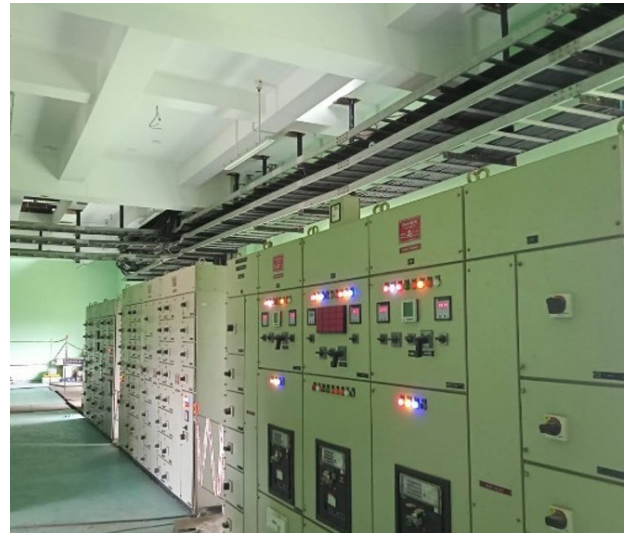
33kV GIS at Birlapur in West Bengal
