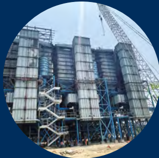
AIR QUALITY CONTROL SYSTEMS
