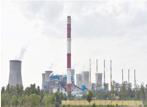
1st Operational Acceptance Certificate for Combustion Modification Package from NTPC Dadri, 2X490 MW
