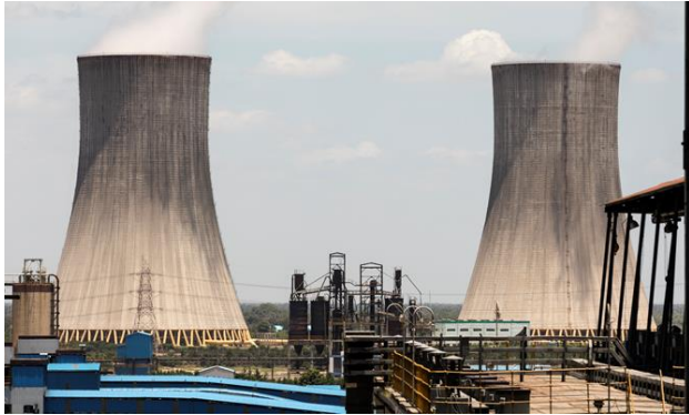
New order win to supply WFGD system to for 2X600 MW Anuppur TPP, from Apollo International Limited for MB Power
