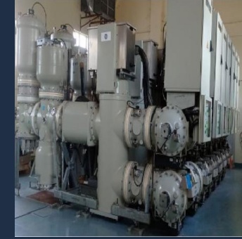
1 X 132kV GIS bay extension for OPTCL Unit VIII at Bhubaneswar
