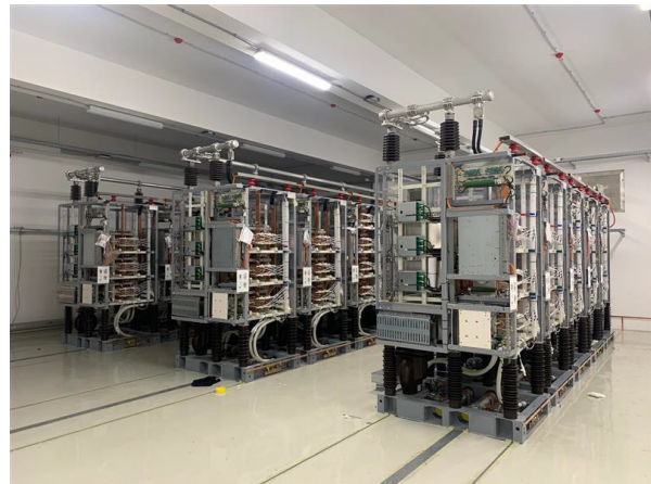
Fig. 3. 100 MVA MMC Delta STATCOM [2]
