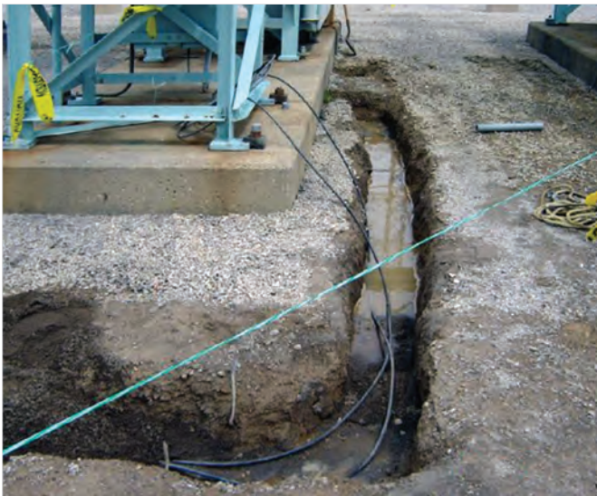
Figure 9. Outdoor communications cable in direct burial application
