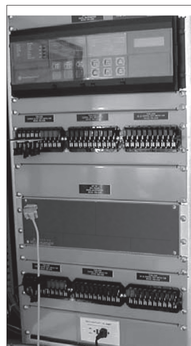
Fig 4. New Feeder Protection and Control Panel Layout.
