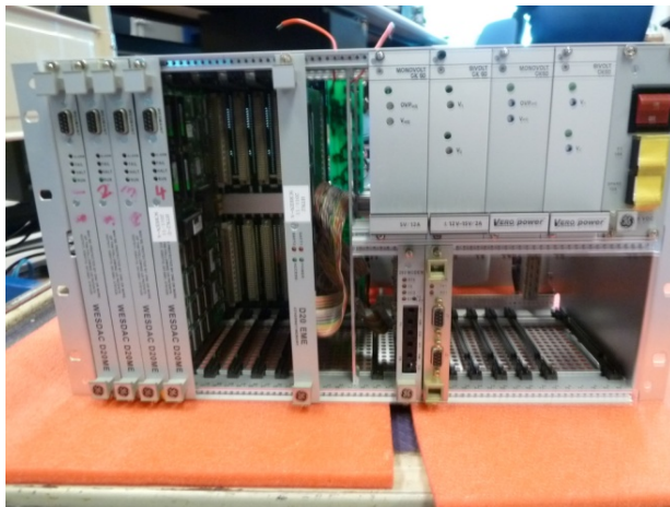
Figure 1: Existing chassis, Front view
