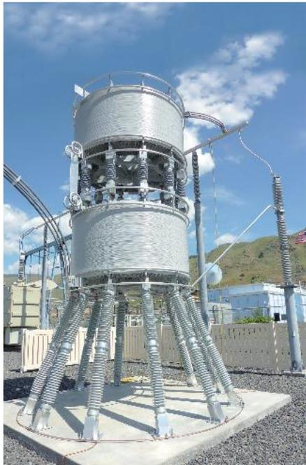
1.1 Current-limiting reactor with seismic design
