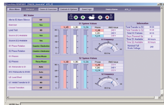
Monitor the status of critical backup assets.
