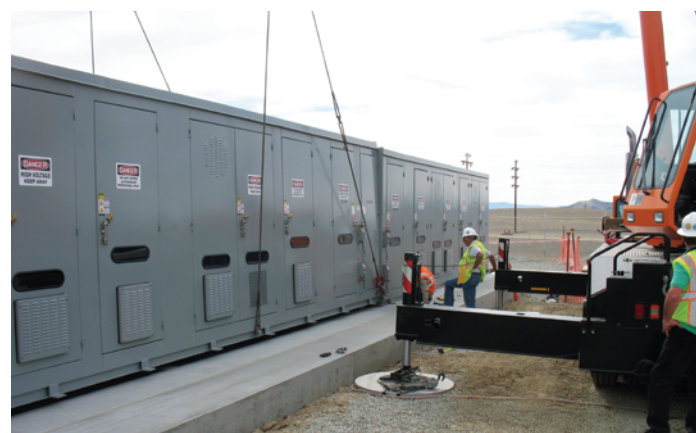
60 MVAR, 38kV, 5-stage 2 section Metal-Enclosed Capacitor Bank being installed at solar plant
