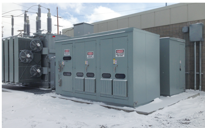
Small Multi-stage Capacitor Banks for commercial and industrial power factor correction.
