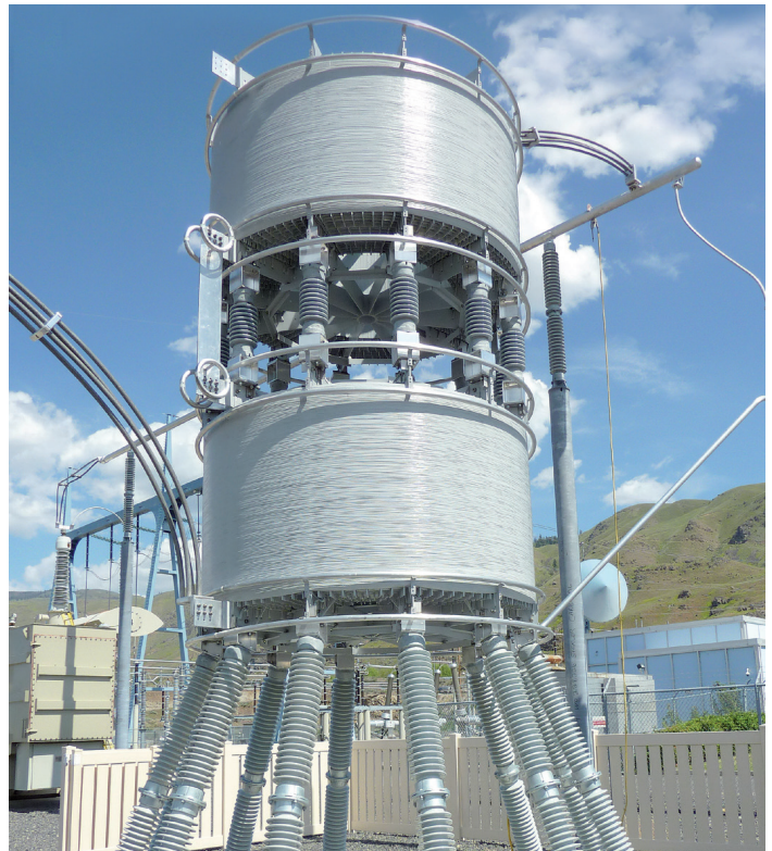
1.1 Current-limiting reactor with seismic design
