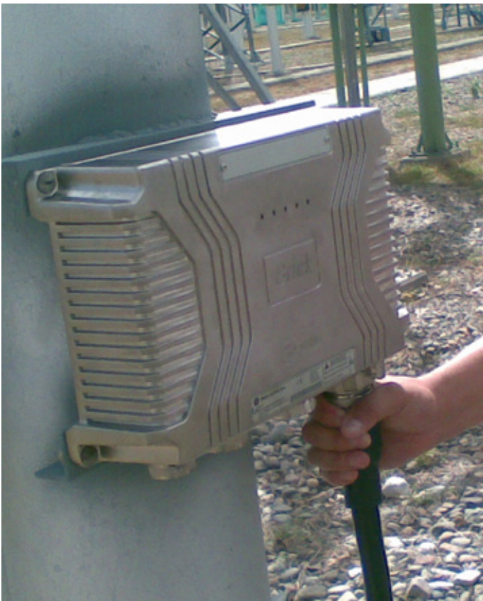
Figure 6A: When installing a process interface unit, operators only need to unscrew the connectorized cables, reducing MTTR time and effort
