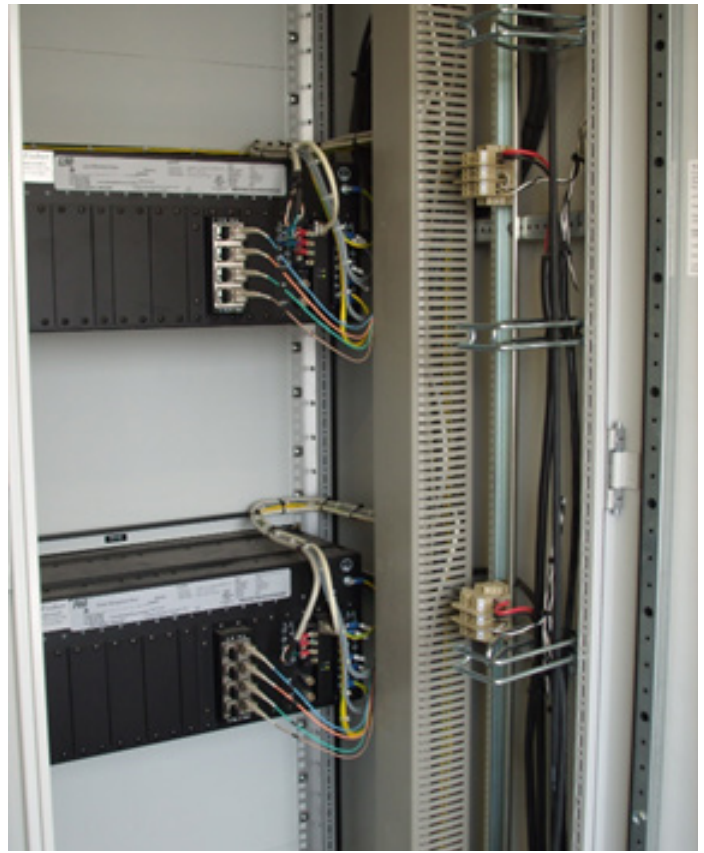
Figure 6B: Installation and/or replacement of a process bus enabled protection and control device is simplified, as only communication wires are connected to the device
