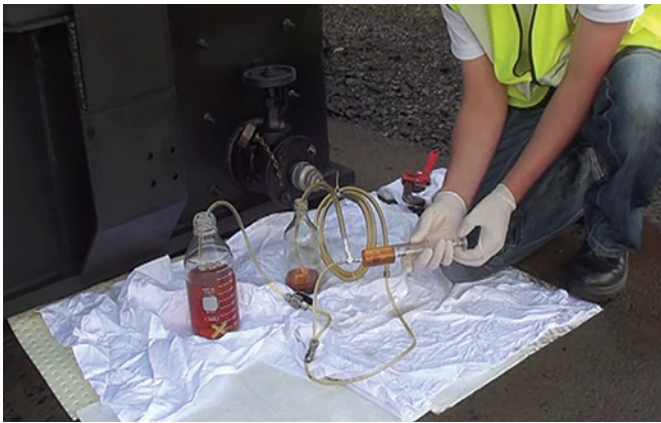
Fig 2: Manual oil sample being taken from a transformer using a gas-tight glass syringe
