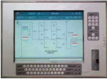
Figure 12. Typical SCADA control monitor
