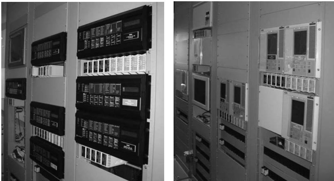
Figure 3. "A" Set and "B" Set Protection
